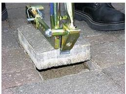
6. Continue removing pavers in the same fashion when the surrounding area is in need of repair. Replace with new paver(s) and sweep sand over the top. Take a piece of 2 x 4, place it over the new paver(s) and hammer with a mallet down the board's length, moving the 2 x 4 around the area. This will act as the compactor did during the initial installation. Fill the joints with sand.
