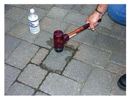
1. In the event pavers on an existing application need to be extracted, pour water around the joint. Then tap the paver to be extracted and the pavers surrounding it. This will help loosen the paver. Remember, if removing a paver from a recessed area, pull pavers from high spot and work down to the recessed unit
