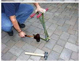
5. When the paver is difficult to extract, stop occasionally and tap the surrounding pavers. The process can be sped up by having one crew member work the PAVER EXTRACTOR while a second taps the surrounding pavers. Many times, there is so much interlock, the surrounding pavers are being lifted along with the paver being extracted.
